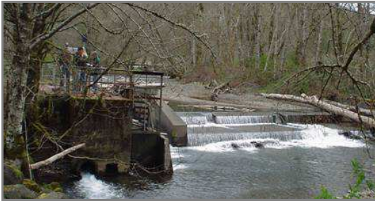
Forks Creek Siphon Intake and Diversion Dam
