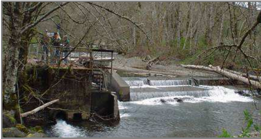
Forks Creek Siphon Intake and Diversion Dam
