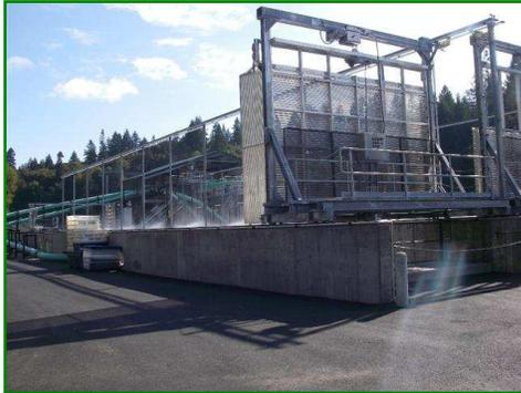
existing large asphalt-lined pond was converted to a series of smaller rectangular concrete ponds equipped with mechanical crowding capability.
