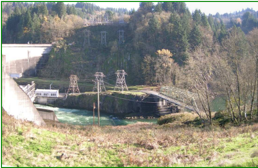
Selected Fish Facility Site
